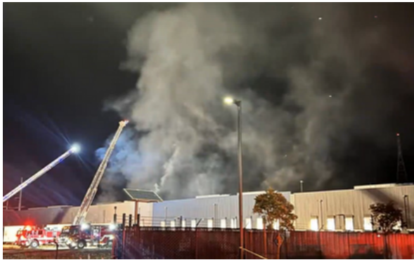
Figure 1: The Otay Mesa energy storage fire burned for nearly two weeks after starting on May 14, 2024 as the result of thermal runaway. Picture provided by San Diego Fire-Rescue.
